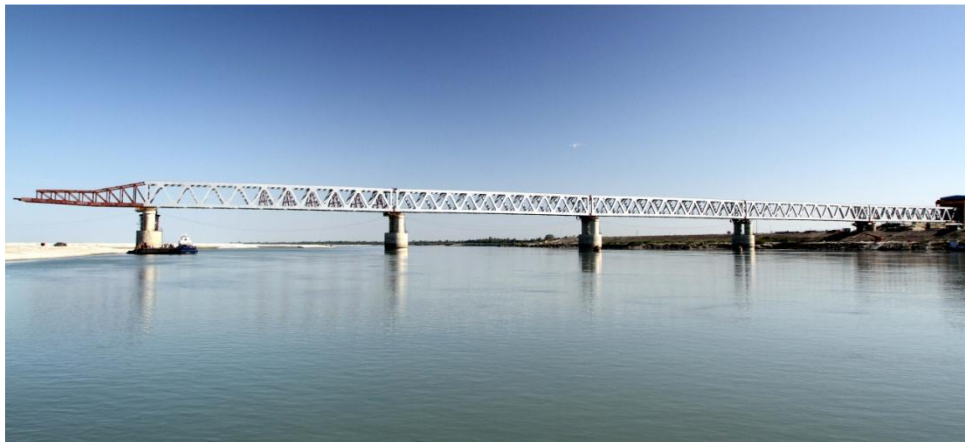
Launching of 5th girder span of Bogibeel Bridge
